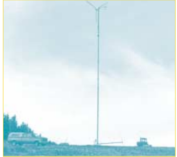
▲ A small stand-alone wind energy system can supply power to both the farm and residence. (Information and photo courtesy of Nor'wester Energy Systems Ltd.)
